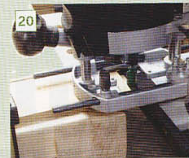
20 The half-lap joints are cut with a router using the side fence
