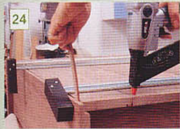
24 The last board is levered tight
