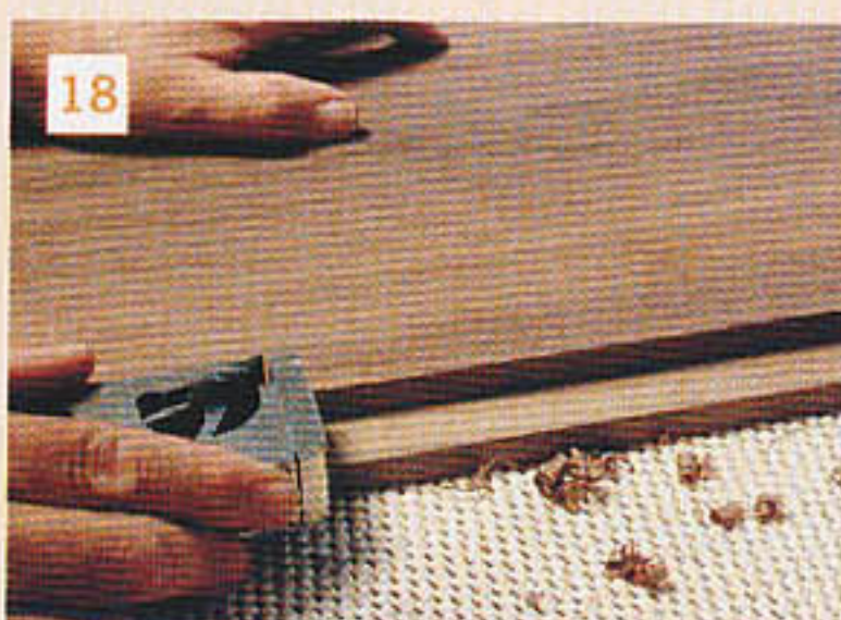
18 Re-establishing the rebate – by hand
