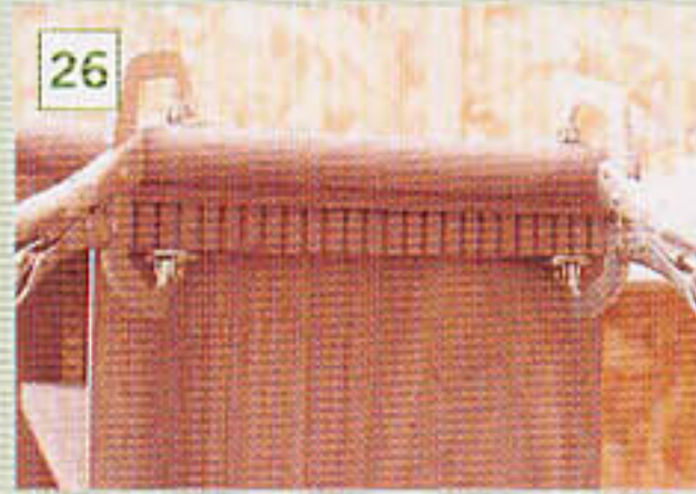
26 Fitting the mouldings...
