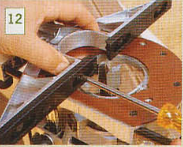
12 A second, deeper recess is cut to clear the shelf studs. While the router is out it is used to cut the rebates for the backboard and bead slats
